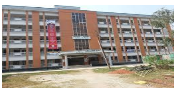
Academic Building (Faculty of Business Administration)
